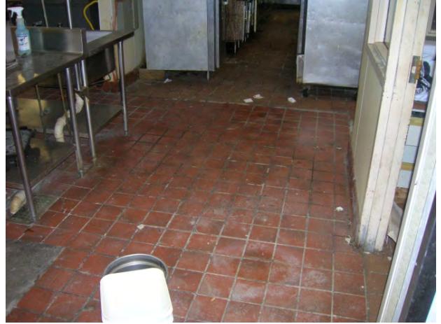
Kitchen – Quarry Tile Flooring
