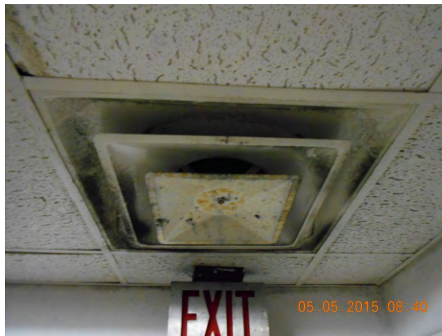
Figure 11 – Supply diffuser mold
