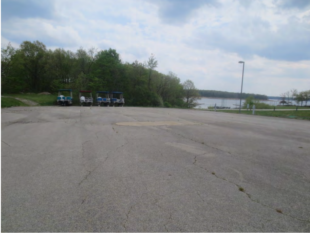
Typical pavement in south parking lot
