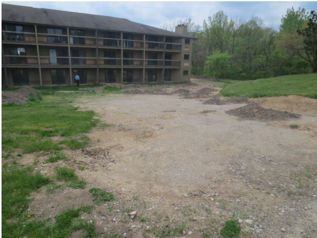
Disturbed landscape area near front of hotel
