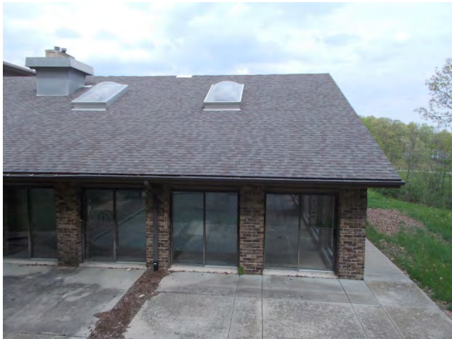
Figure 21 – Roof over Pool Area
