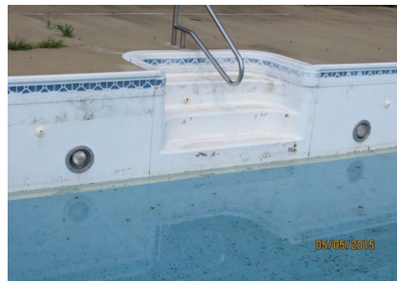
Figure 56 - Swimming Pool – Recessed with Gasket Fixture
