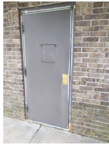
Figure 38 – Hollow-Metal Door without Hardware
