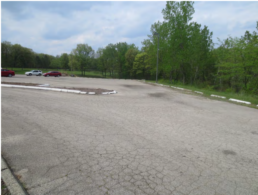
Typical pavement - north parking lot area pavement
