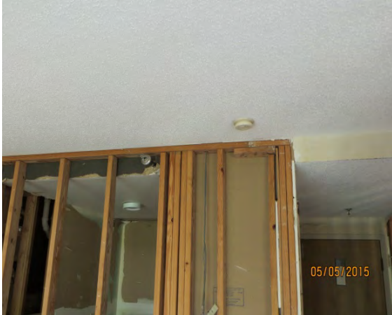
Figure 47 - Typical Ceiling Mounted Smoke Detector
