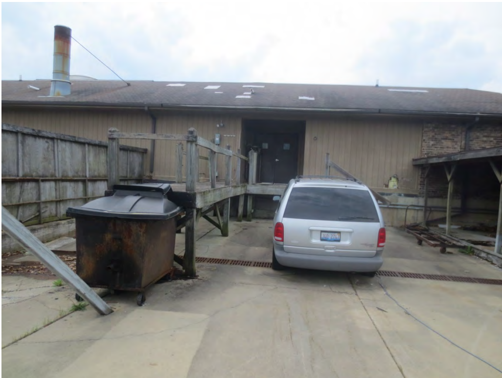
Loading dock area; note wooden dock platform
