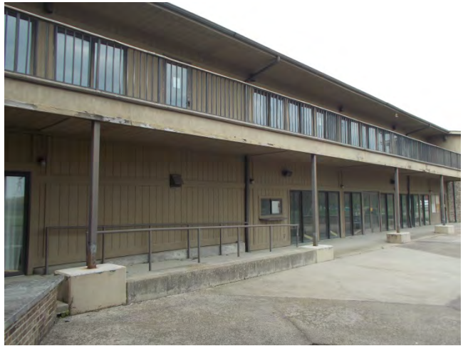
Note Exterior Ramp
