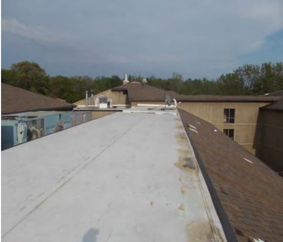
Figure 71 - Existing Cable TV Dish Antennae
