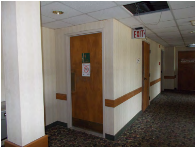
Toilet Room Access
