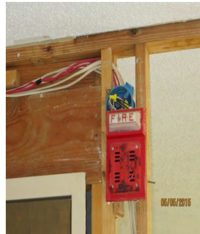
Figure 70 - Typical Audio Visual Alarm
