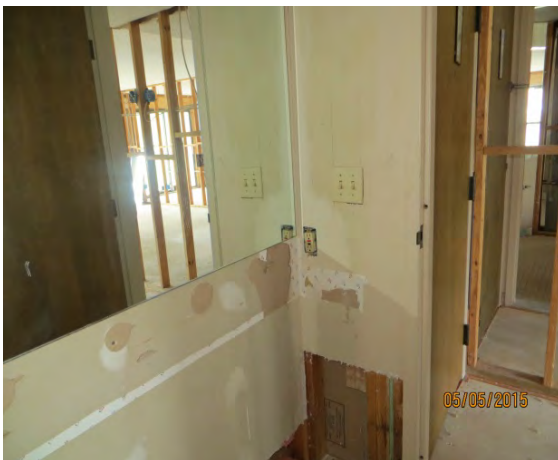
Figure 45 - Typical Bathroom Wall
