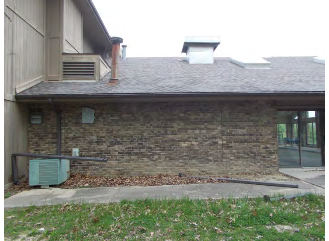
Figure 16 – Hotel Entrance Wall
