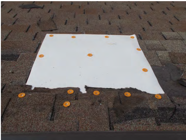
Figure 25 – Roof Patching
