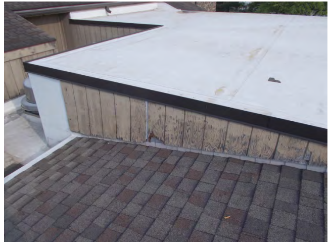
Figure 22 – Various Roof Conditions
