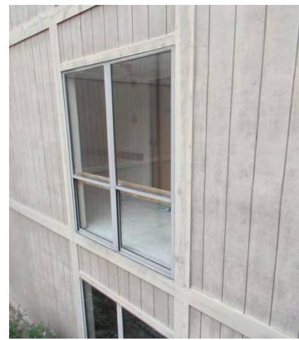
Figure 32 – Typical Fixed Window
