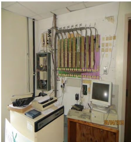
Figure 62 - Existing Main Telephone Distribution System
