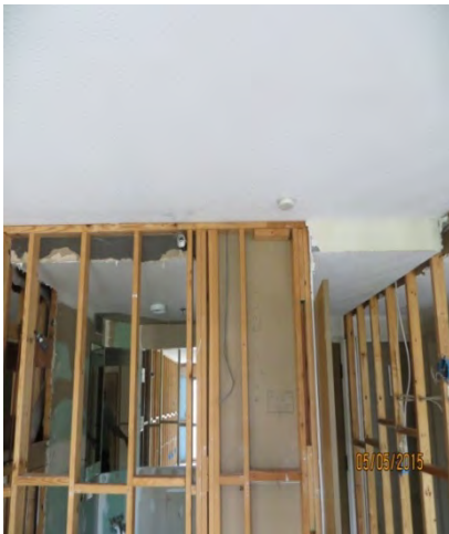
Figure 69 - Typical Smoke Detector in Guestroom
