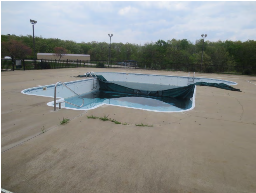
Pool Area concrete
