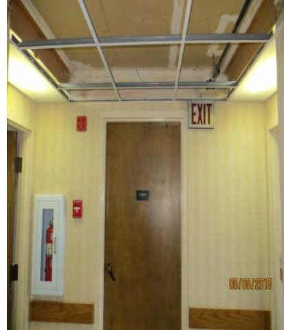
Figure 68 - Existing Manual Pull Station
