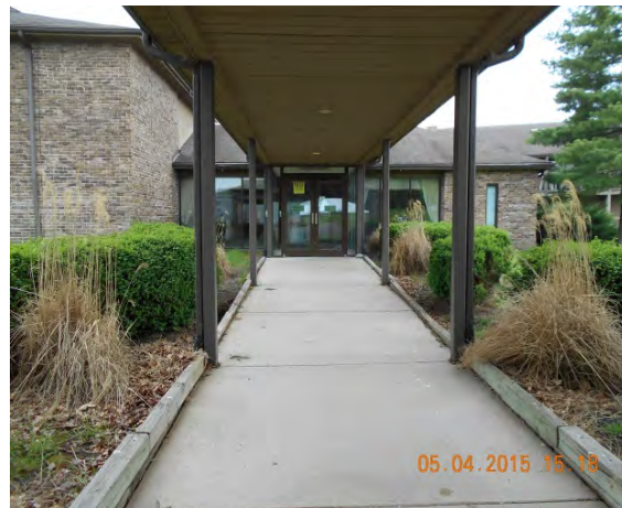
Figure 20 – Entry canopy to main lobby
